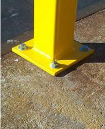
Welded baseplate provides maximum rigidity for post installation
