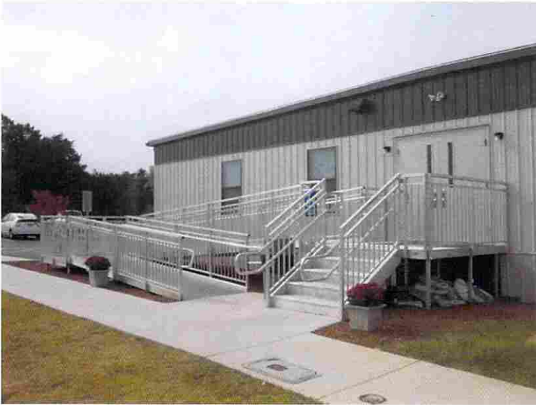
TYPICAL RAMP INSTALLATION
