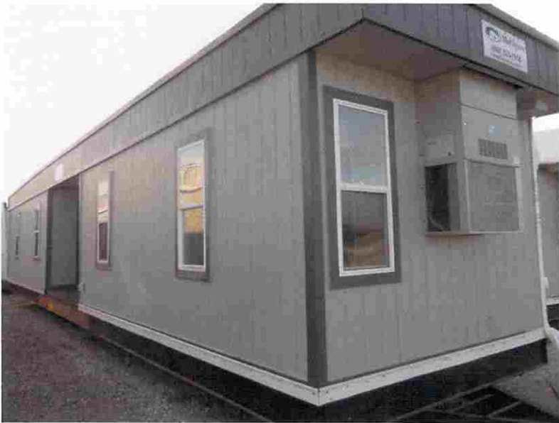
UNIT IN STORAGE (FRONT)
