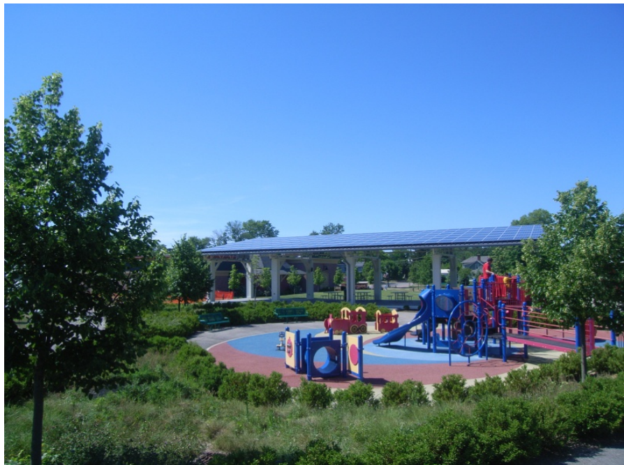
Solar Pavilion at Village Green Park, completed in 2012, funded by ARRA grant funds
