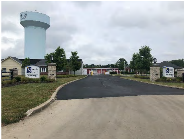
Simply Self Storage located on Woodcutter Drive south of Home Road and east of Ale Wine & Spirits
