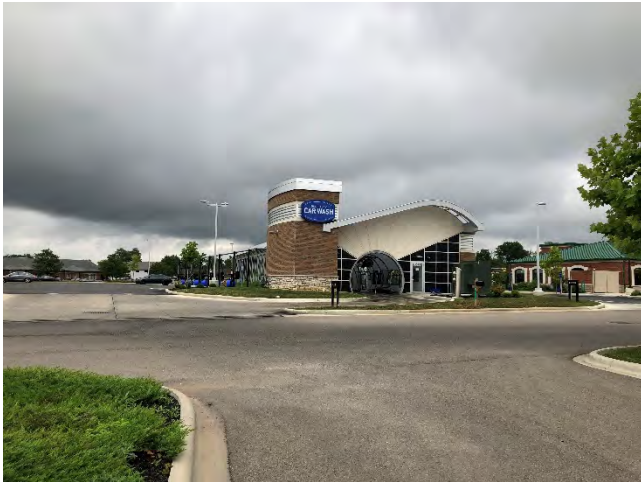
Blue Sky Car Wash located north of WesBanco and east of the Target Parking Lot
