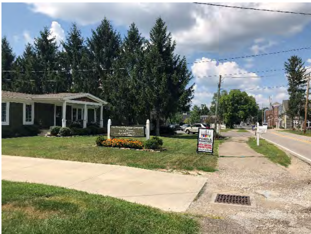
The Powell Painting Company located on the west side of South Liberty Street, view facing north on Liberty
