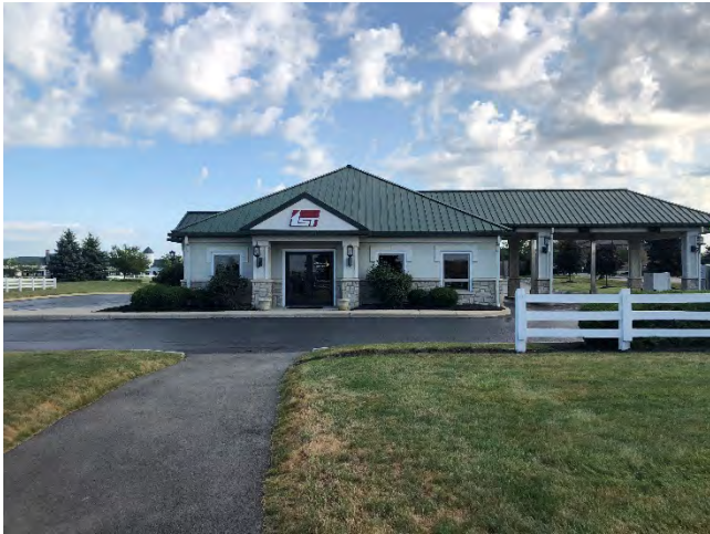
First Citizens National Bank located on the northeast corner of Sawmill Parkway and Powell Road south of Raising Cane’s
