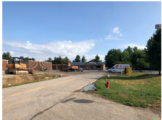
Cardinal Self Storage located on the west side of Industrial Park Place north of Gerber Glass and Collision and west of Locker Soccer Academy
