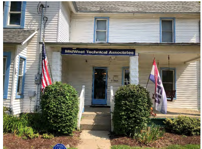
Midwest Technical Associates located on the north side of West Olentangy directly west of the train tracks, east of Milano Florist
