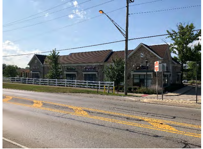
Powell Retail Center located on the southwest corner of West Olentangy and Murphy Parkway east of Handel's Ice Cream
