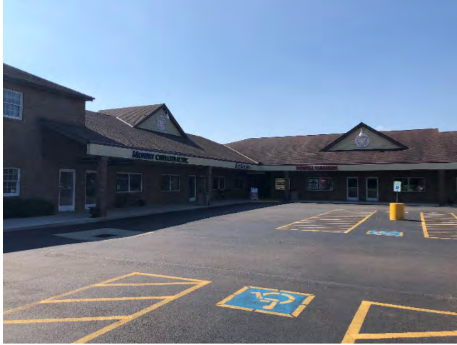
Liberty Square Shopping Center (south side of Grace Drive across from Grace Plaza) showing Mowry Chiropractic and Powell Cleaners
