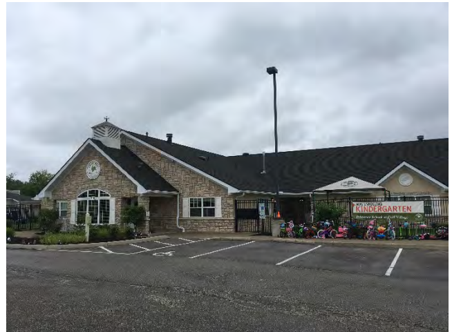
Primrose School located south of Enchanted Care Kingdom on Moreland Street
