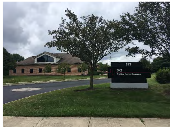
Building Control Integrators located on the west side of N. Liberty Street south of North Powell Office Condominiums
