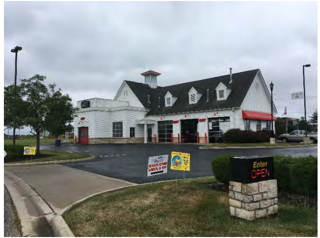
Ron's Express Car Wash located on Moreland Street, east of the Golf Village shopping center and south of the empty lot
