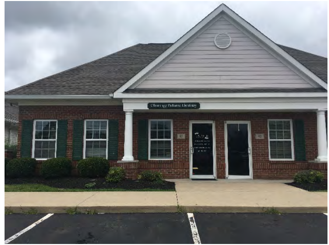
Olentangy Pediatric Care located in North Powell Office Condominiums
