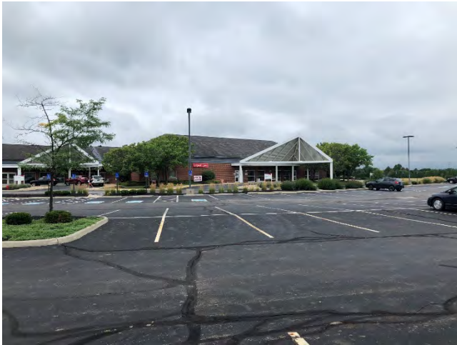
View of Urgent Care and parking lot
