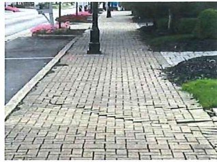
Existing Paver Sidewalk - 1
