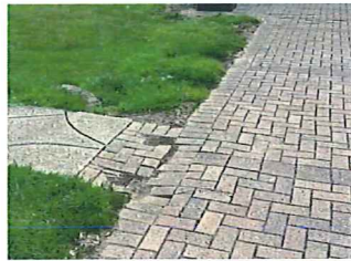
Existing Paver Sidewalk - 2
