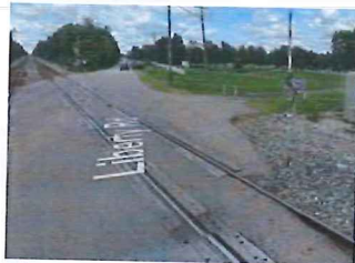
Liberty Road Northbound at Railroad
