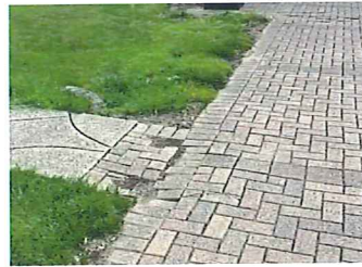
Existing Paver Sidewalk - 2
