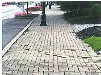
Existing Paver Sidewalk - 1
