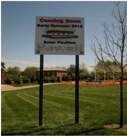
Solar Pavilion Construction
