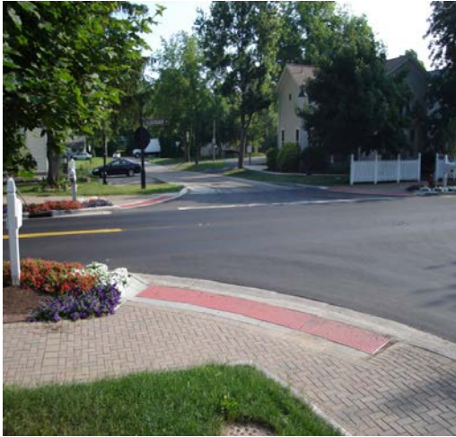
Road, curb and handicap ramps
